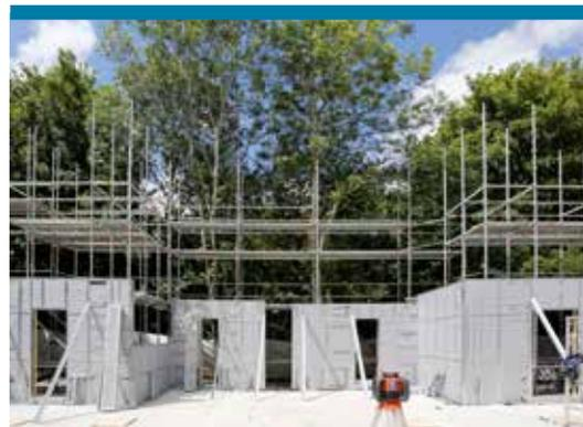
Panelised light-gauge steel frame construction
