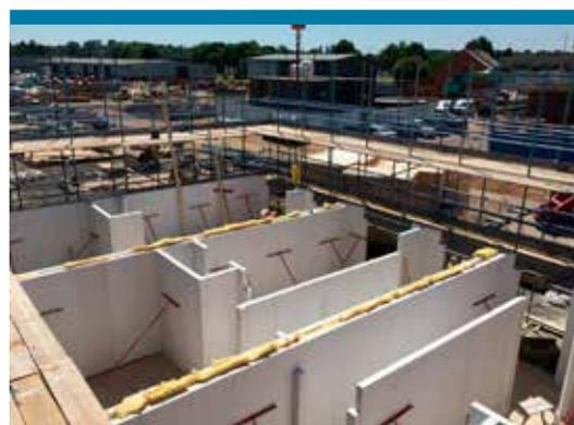
Installation of storey-height aircrete panels
