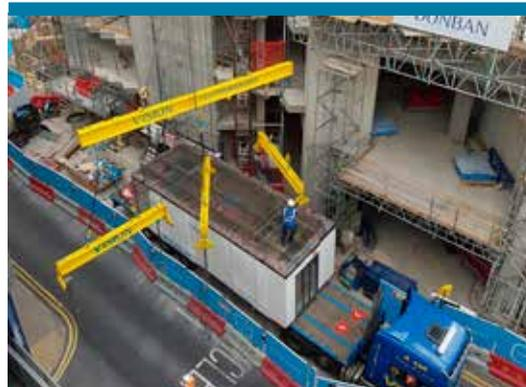
Fully-fitted volumetric modules delivered to site
