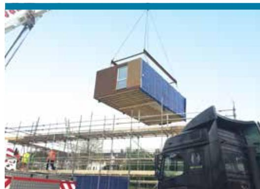
Installation of fully-finished volumetric modules
