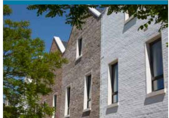
Brick facade to closed-panel timber frame houses
