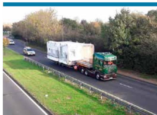
Two fully-fitted volumetric modules in transit to site
