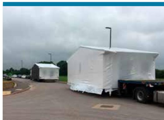
Fully-finished volumetric modules in transit to site
