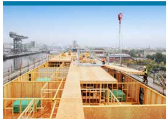
Erection of open-panel timber frame in Glasgow
