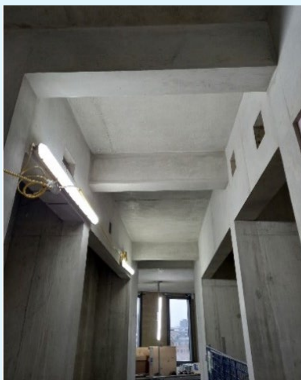
FIGURE 1 – Lobby slab/beam with Elder Yard core
